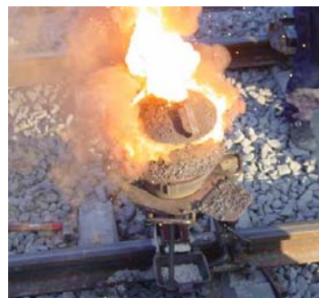
Welding railroad track with Thermite
